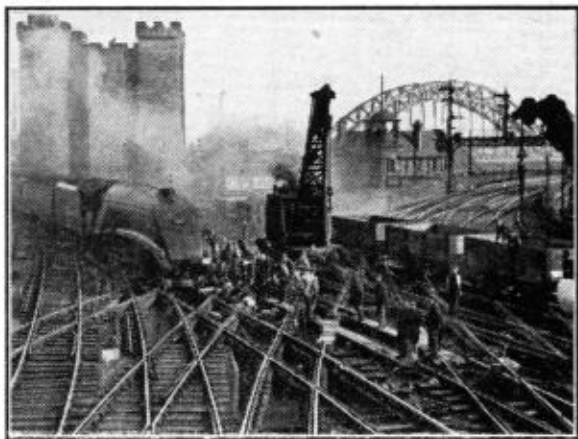
An up express from Edinburgh picks its way along the only track left open during the renewal of the crossings near the High Level Bridge at Newcastle. British Railways Official Photograph.
