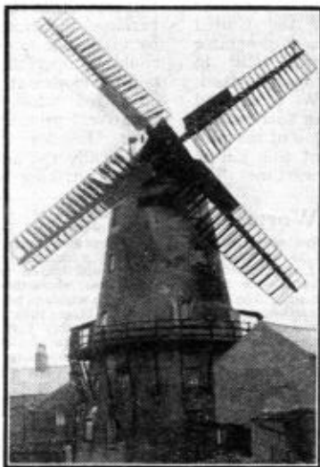
Windmill sails are cumbersome and less efficient than the streamlined blades of a modern aero-generator. This old windmill is at Thornton-le-Fylde, Lancashire.
