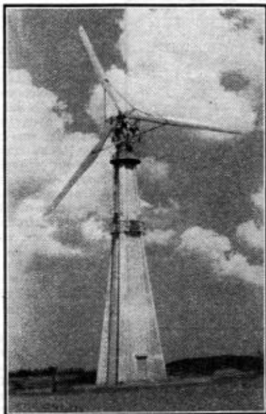
A three-blade wind turbine such as this can attain a very high speed and is particularly suitable for generating electric power.
